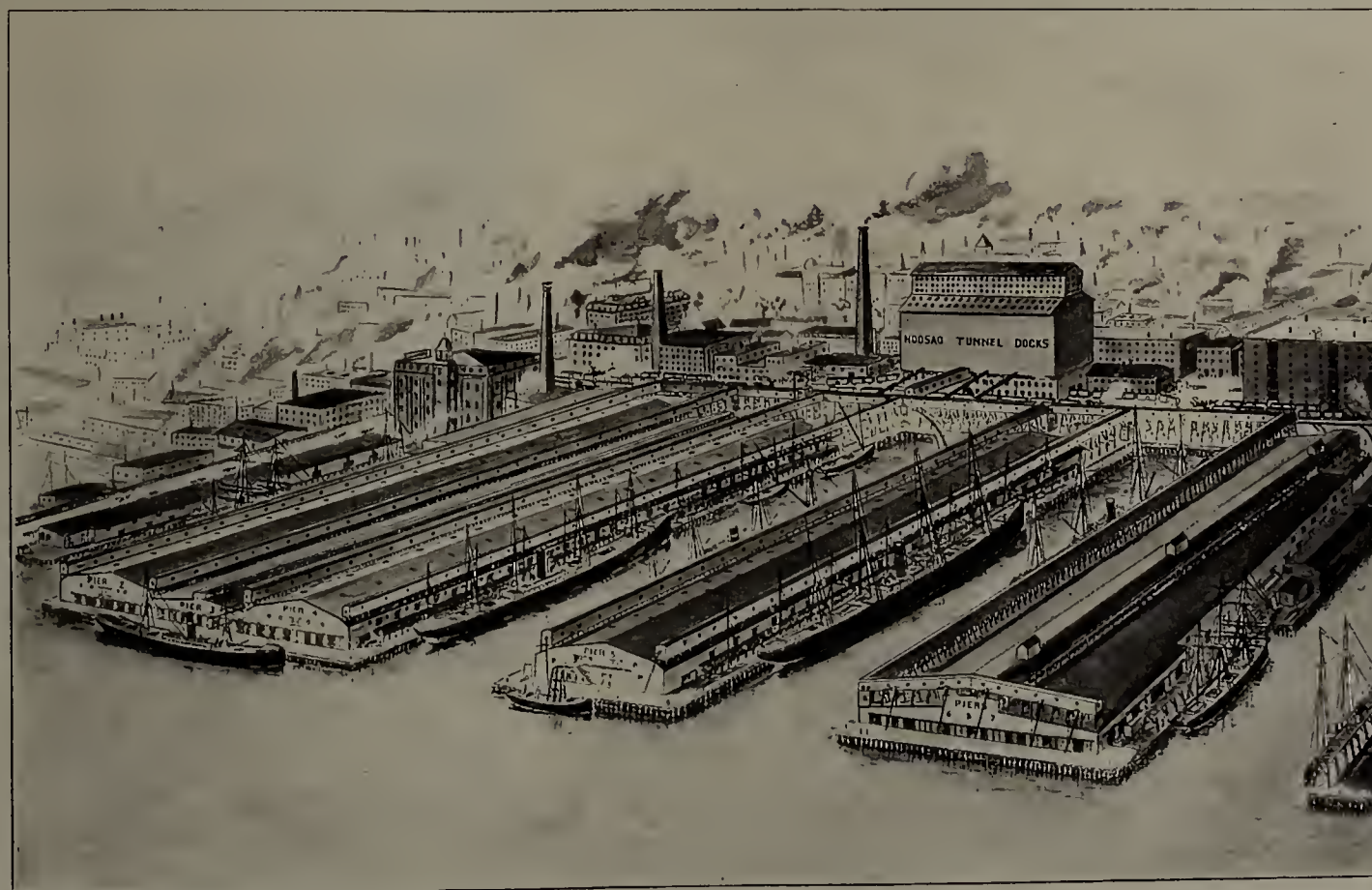
HOOSAC TUNNEL DOCKS AND ELEVATOR OF THE FITCHBURG RAILROAD, Charlestown Water Front of the City. Five piers; elevator of 600,000 bushels capacity; ample water at all stages of the tide; stone and iron warehouses; hydraulic lifts and grain conveyors; electric hoists and lights throughout. Foreign Freight Office, 204 Chamber of Commerce.
